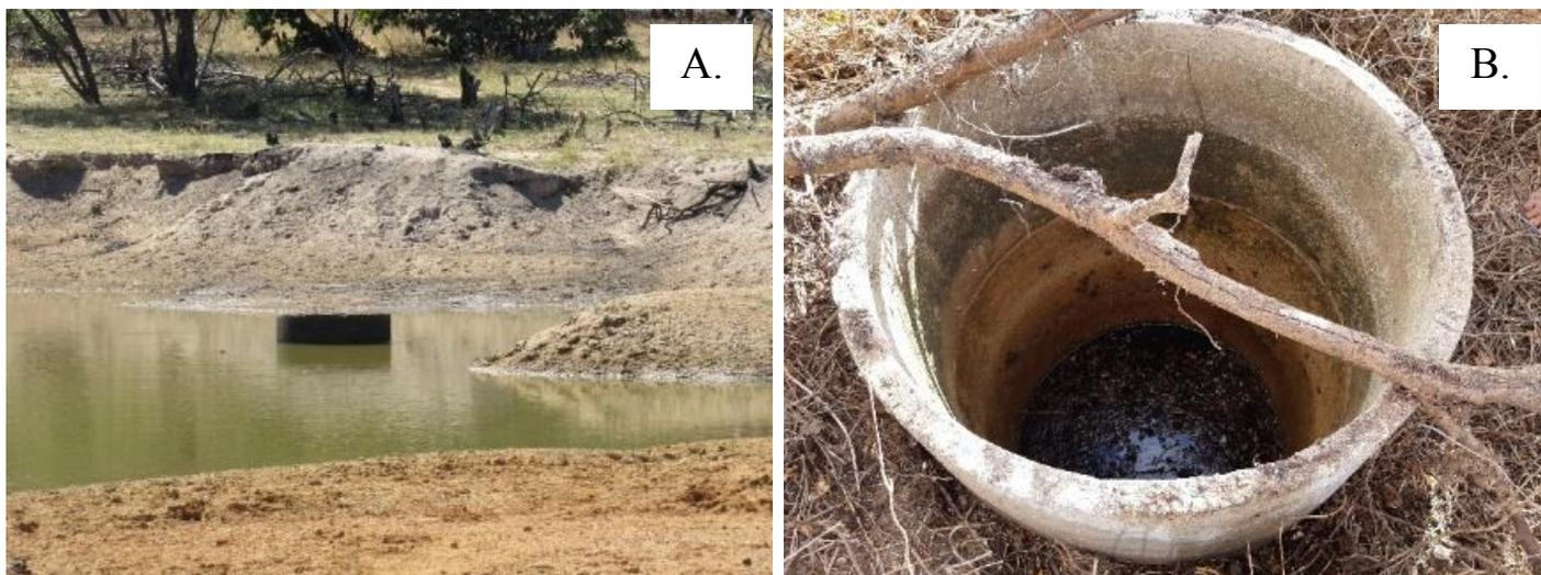
**Figure 4.** Problems related to increase in concentrations of total suspended solids in shallow wells of the analyzed underground dams: CD dam (A), TP dam (B).
