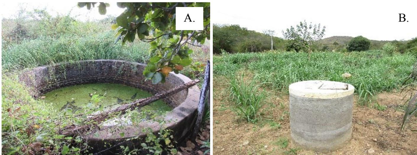
Figure 2. Examples of shallow wells within underground dams: C-T1 (A), CE-RF1 (B).
